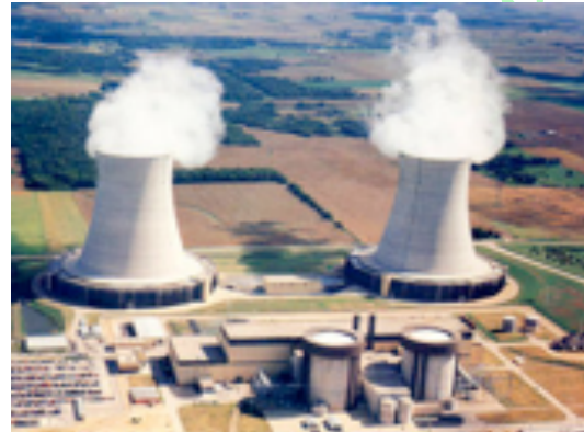
A Nuclear power plant (Wikipedia.org)
